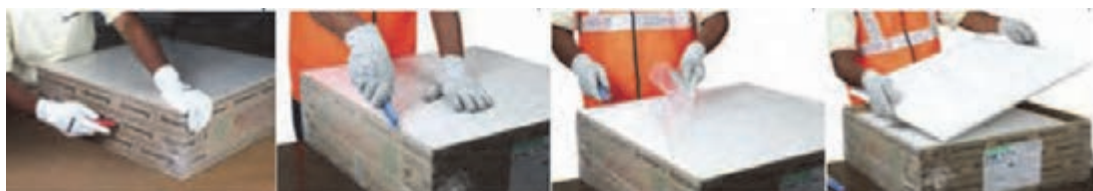
Wrong box opening method
