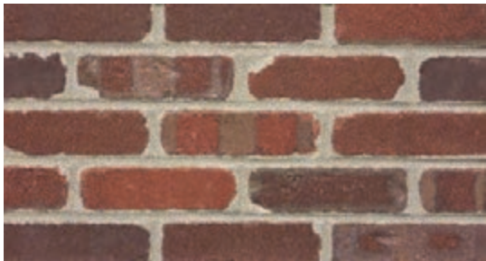
Standard 3/8" Mortar Joint
